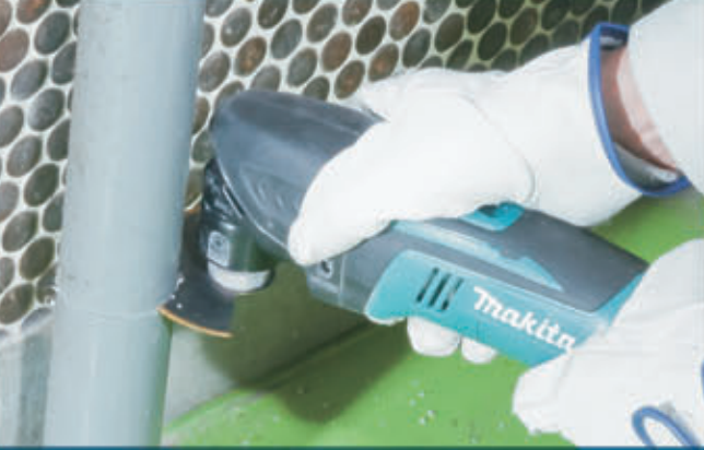
Cutting PVC, FRP pipes
