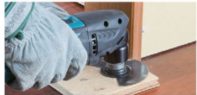
Wood flush cutting
