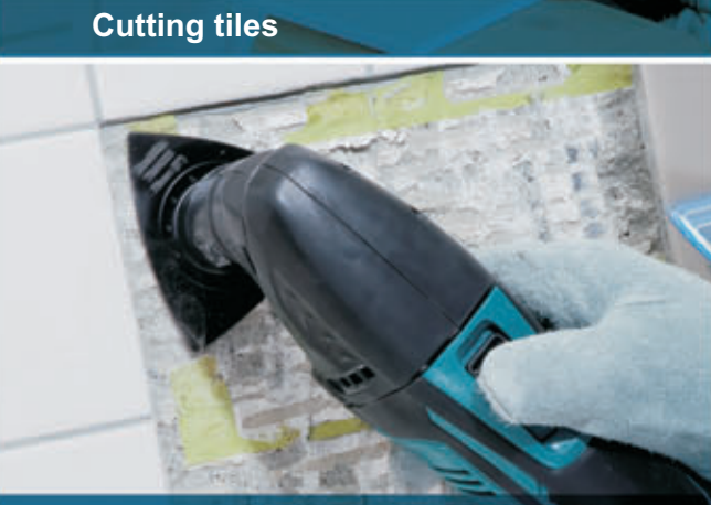
Removing mortar, tile adhesive
