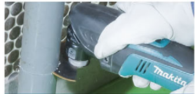
Cutting PVC, FRP pipes
