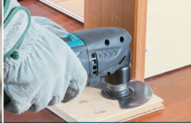
Wood flush cutting
