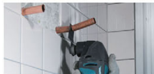
Cutting copper pipe
