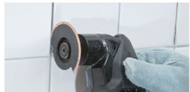
Routing joints on wall tiles
